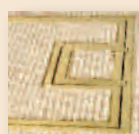
Thick carpet installation using 1/2" brass edging on cover
